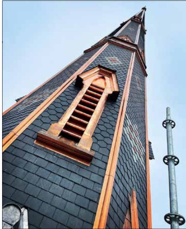
Construction work at Central Presbyterian Church in Cambridge, Ont.
